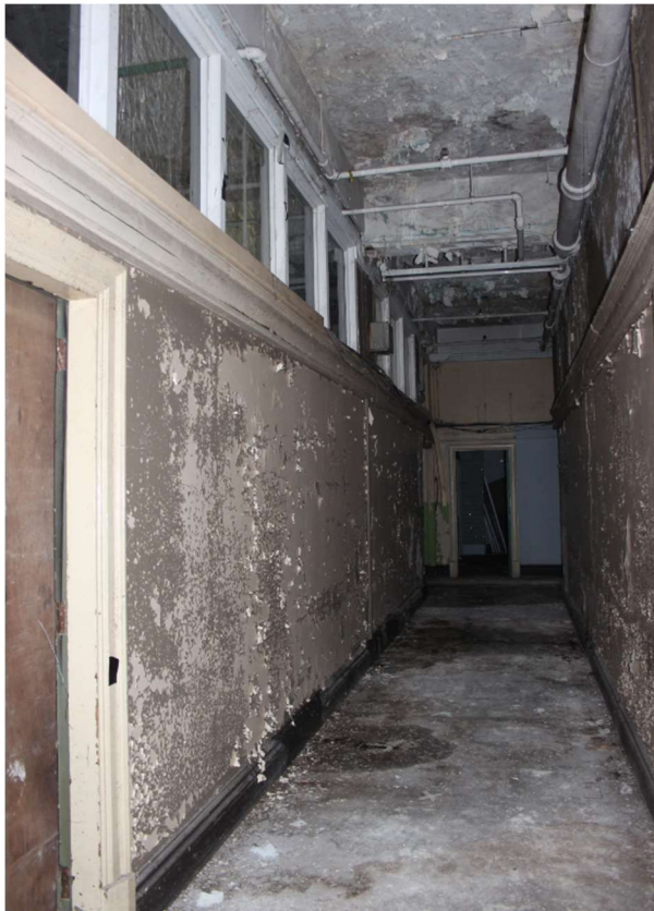
Figure 4: View of internal joinery elements within the front three bays of factory No. 2, including architraves, skirtings and timber panelling.
