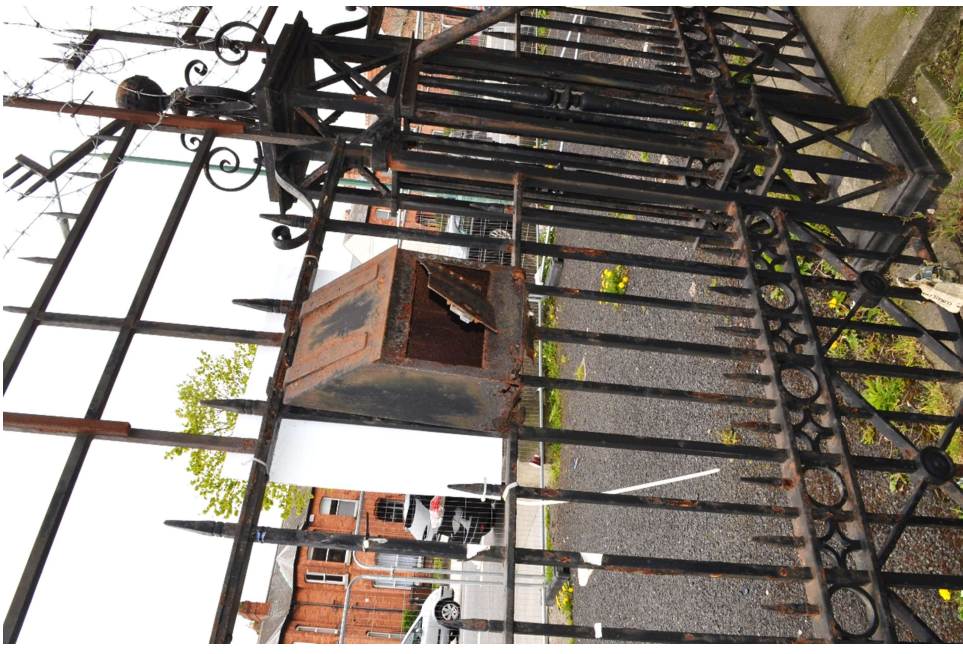
19. View of the entrance gate to the east of Block A
