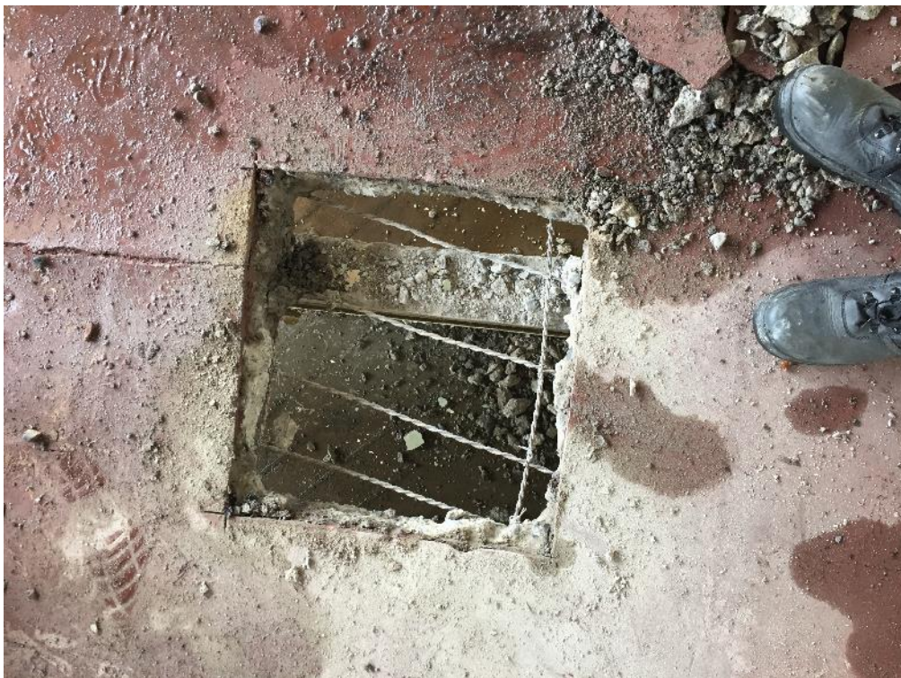
Photo 27: Level 3 reinforcement
