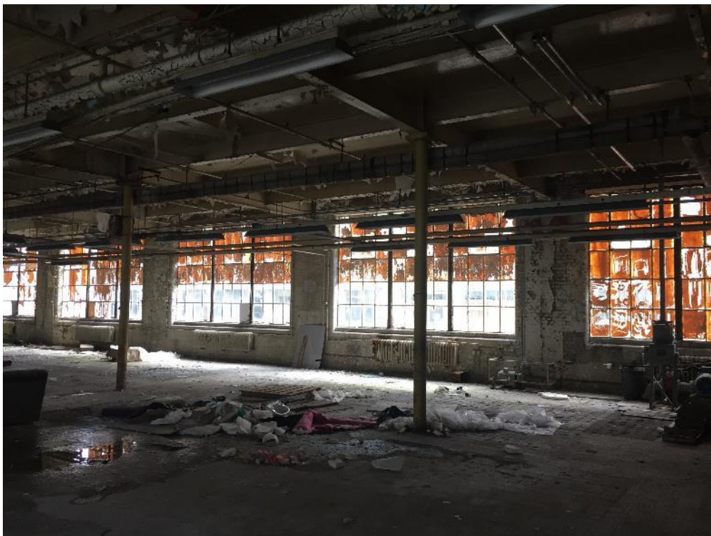
Photo 2: Original Building Condition
