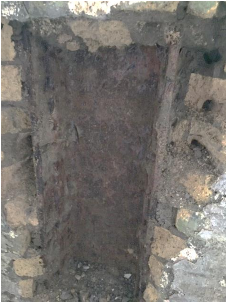
Photo 19: Embedded Steel
