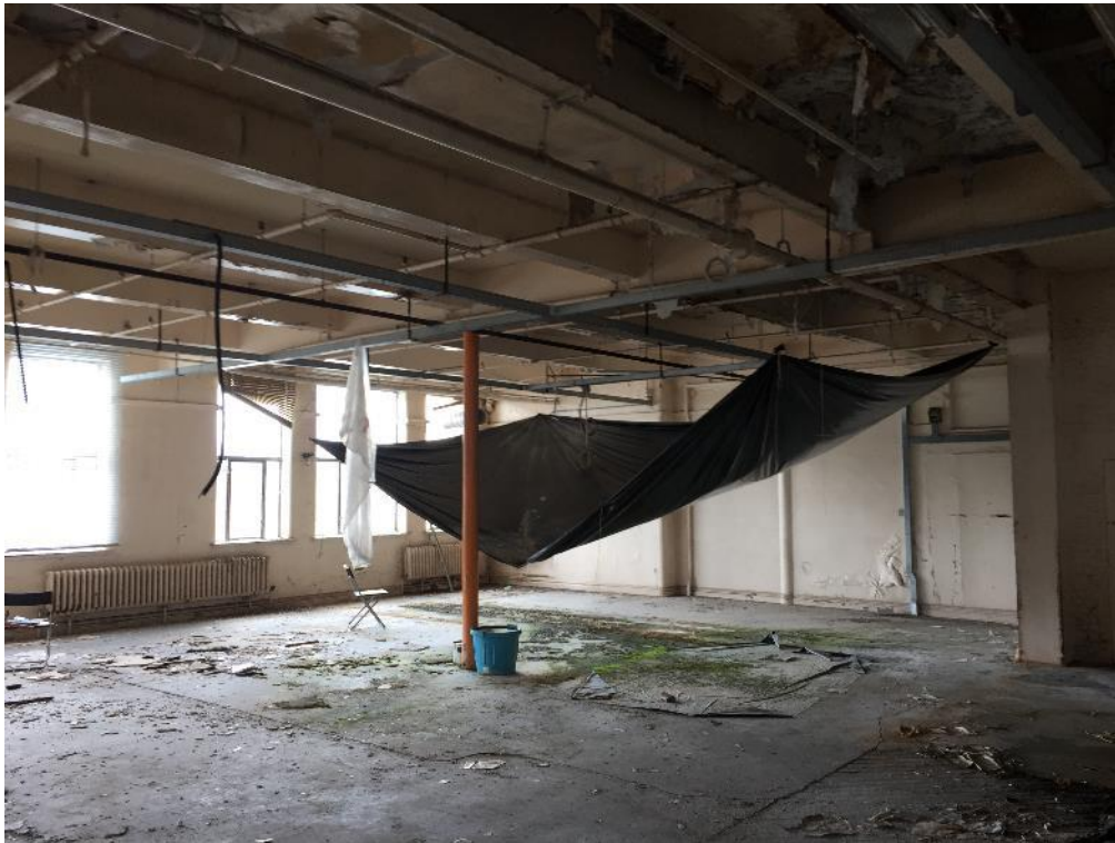
Photo 5: Original Building Condition
