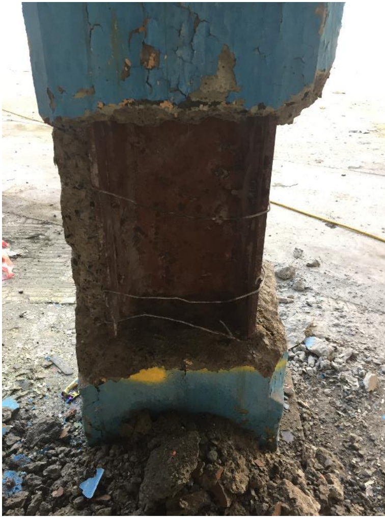
Photo 20: Embedded Steel
