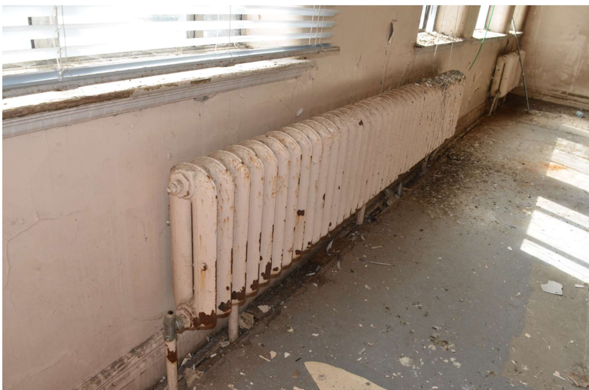
Figure 9: Cast-iron radiator.
