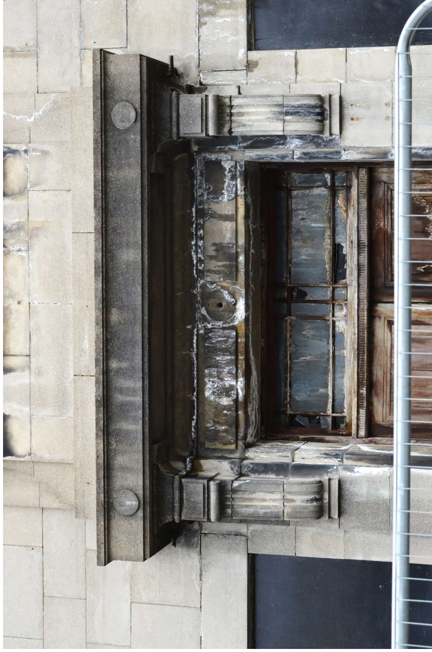
14. View of the door surrounds and over-light to the main entrance of Block A
