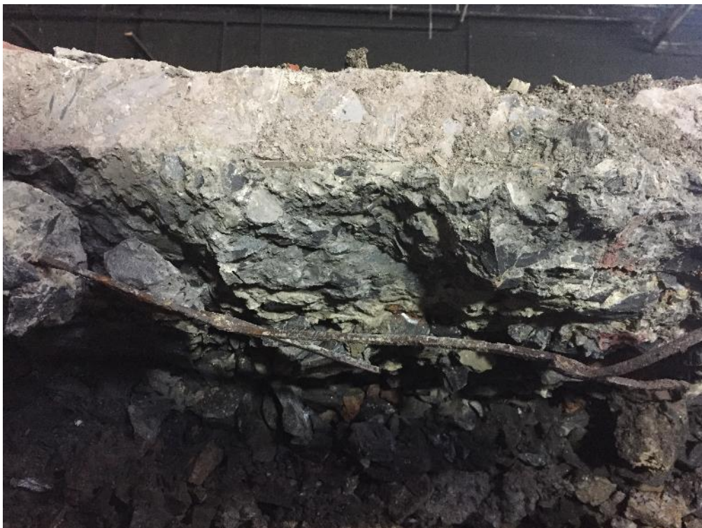
Photo 22: Ground Floor Slab
