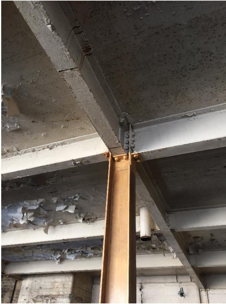
Photo 13: Level 2 column (1930's section) with level 3 beams
