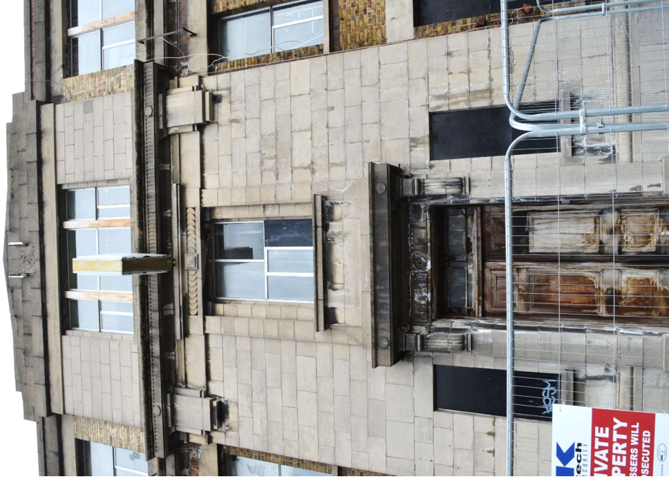
13. View of the central breakfront entrance bay to the southern façade of Block A
