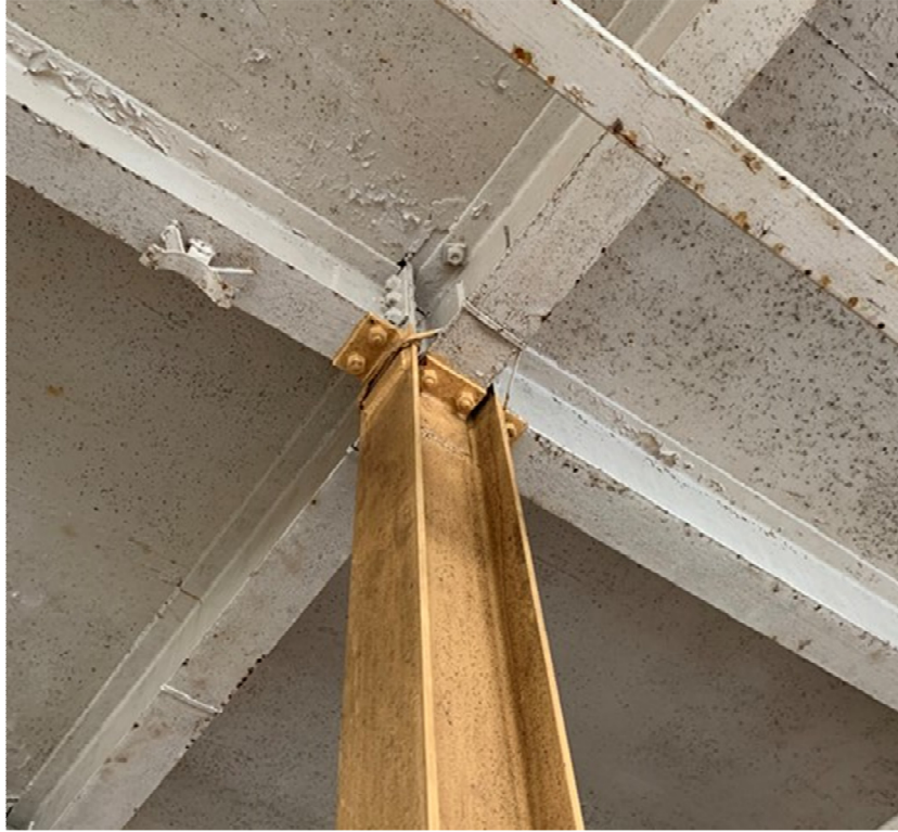
Plate 6: Steel beams and columns
