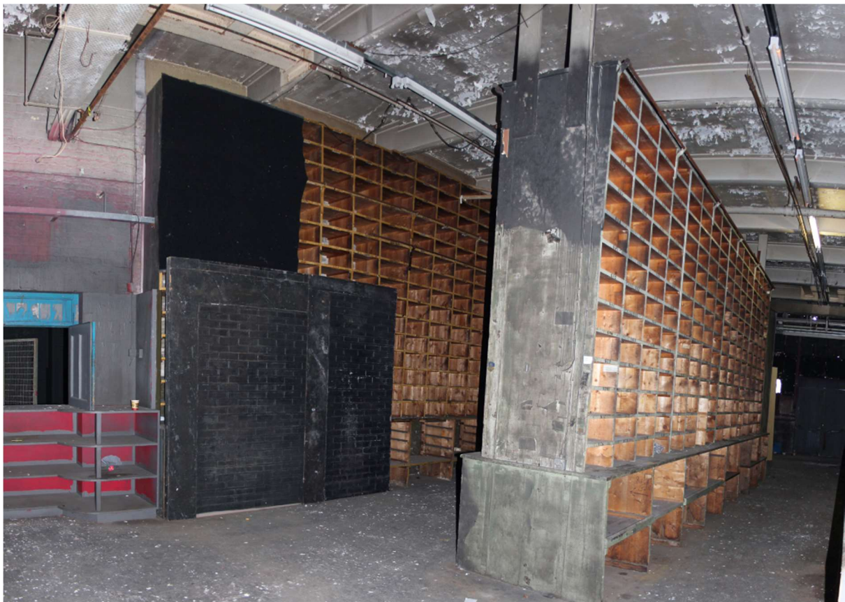
Figure 11: Timber cubby-hole storage in Room G5.
