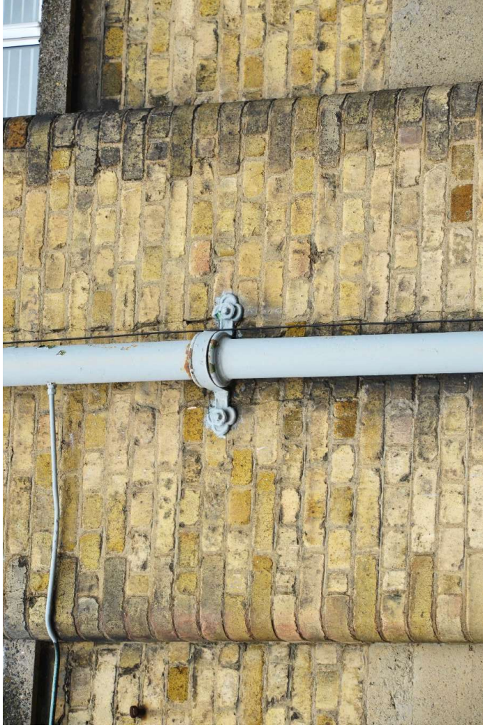
28. Downpipe on the eastern elevation of Block A
