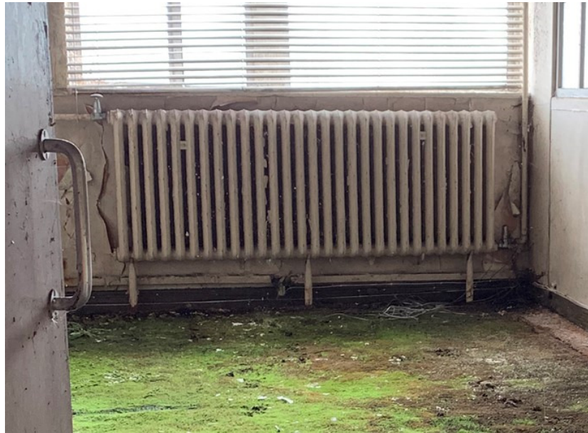
Plate 18: Cast-iron radiator
