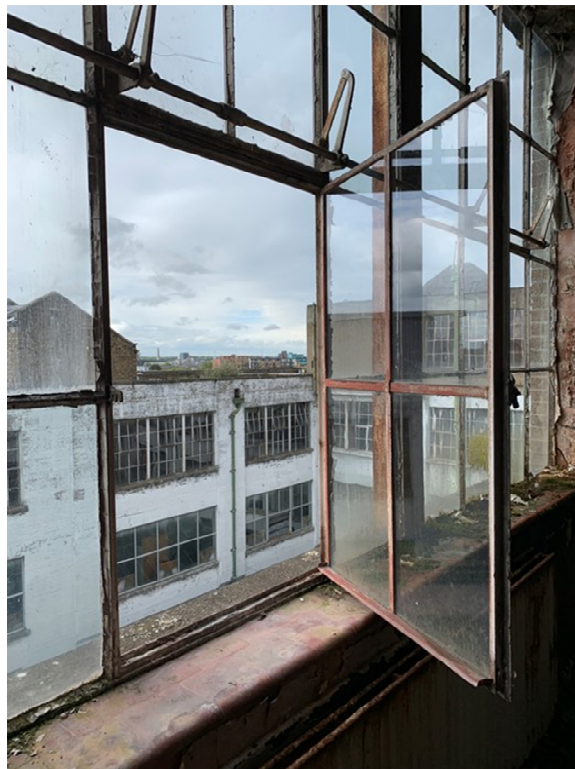
Plate 7: Steel windows and opening mechanisms
