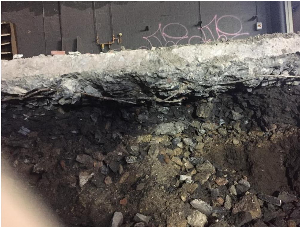
Photo 21: Ground Floor Slab
