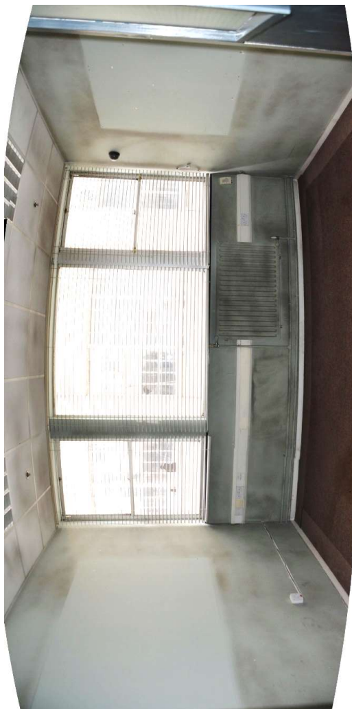
6. Office – Ground Floor Level
