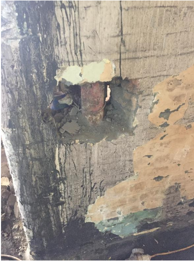
Photo 16: Embedded Steel
