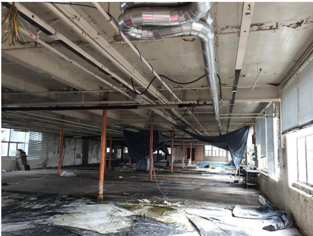
Photo 4: Original Building Condition
