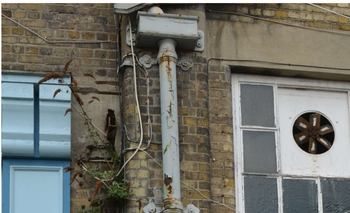
Figure 7: Cast-iron hopper, downpipe and straps.
