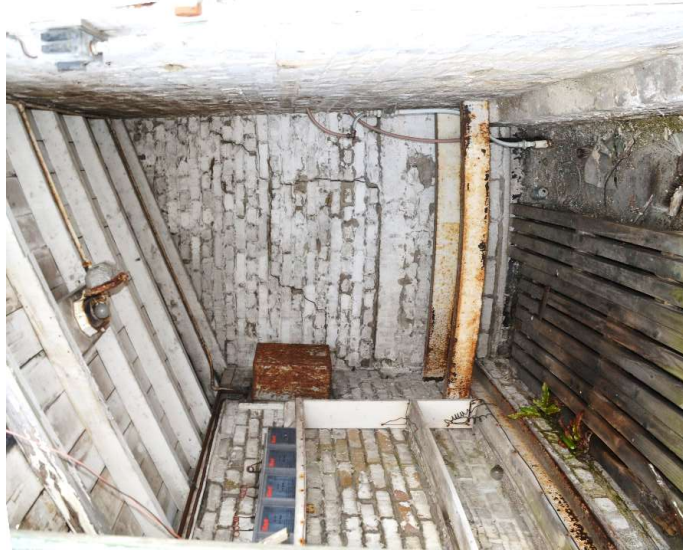
5. Northern room of R2
