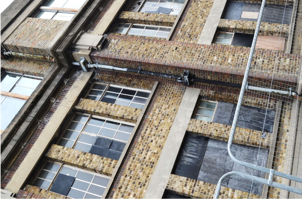
12. View of the rainwater goods on the front façade of Block A
