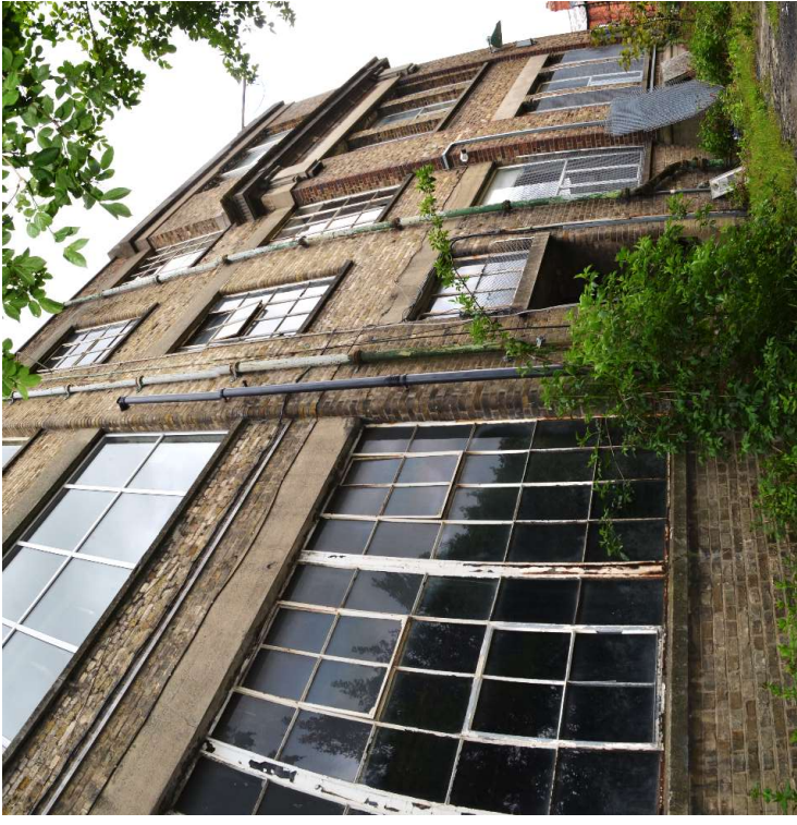
62. Oblique view along the western elevation of Block A
