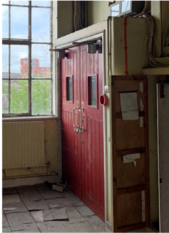
Plate 10: Doors and door closers
