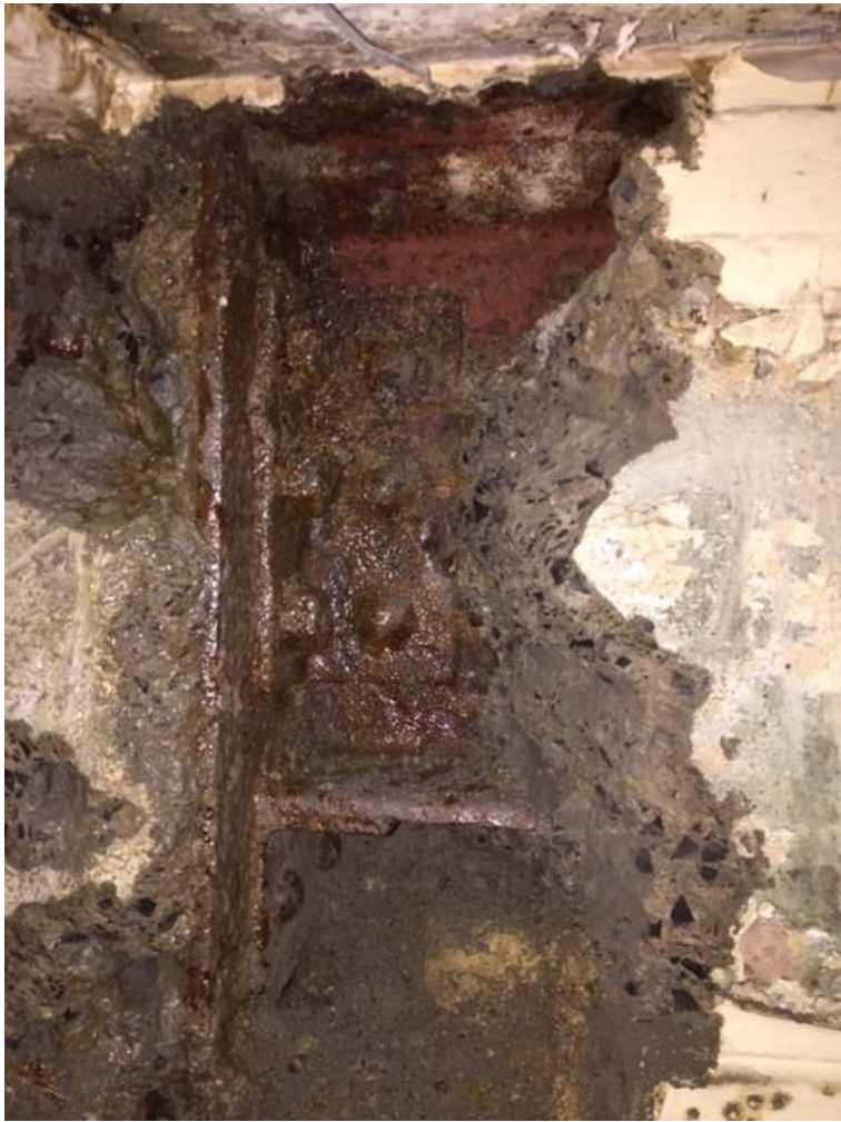
Photo 18: Embedded Steel
