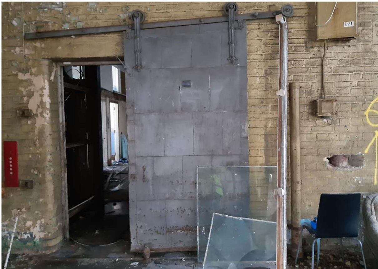
Figure 5: Sliding industrial steel door in Room G.11.
