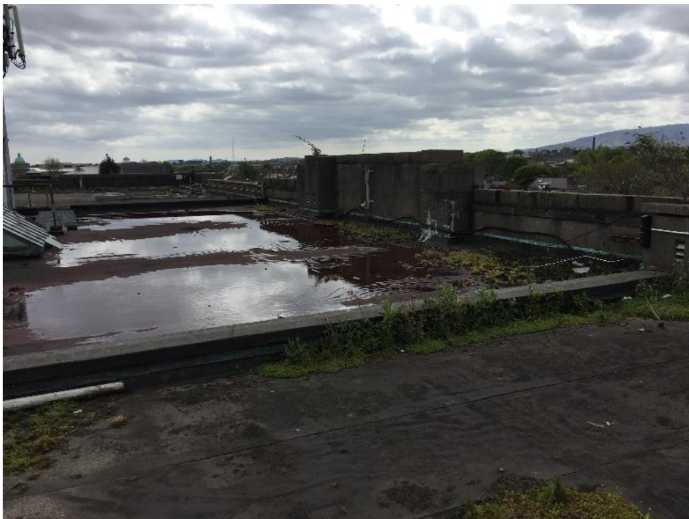
Photo 9: Original Building Condition
