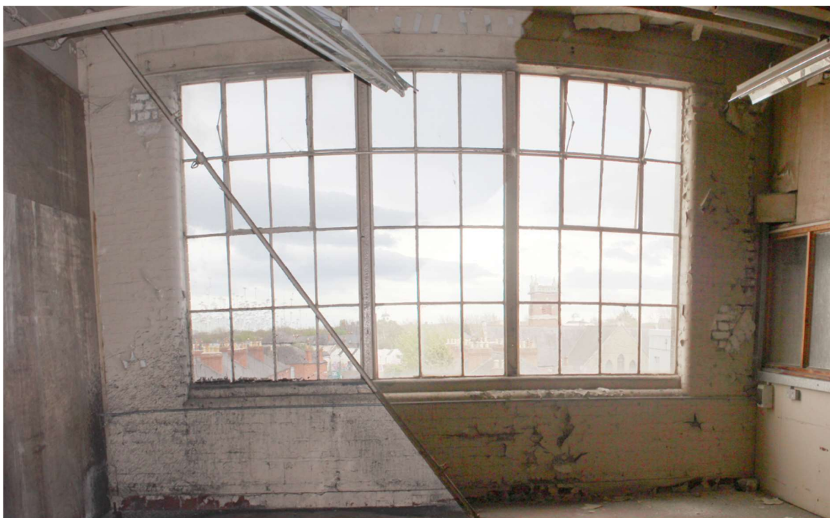
Figure 6: Original steel multi-pane window.
