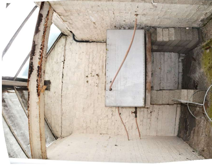
6. Southern room of R2
