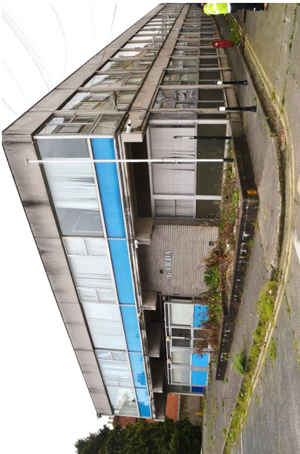
43. View of the northern and western elevations of Block C
