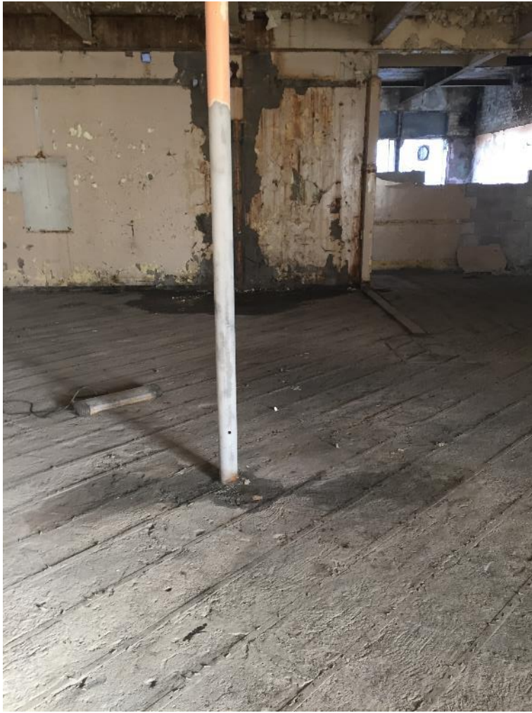
Photo 14: Level 2 column for 1920's section
