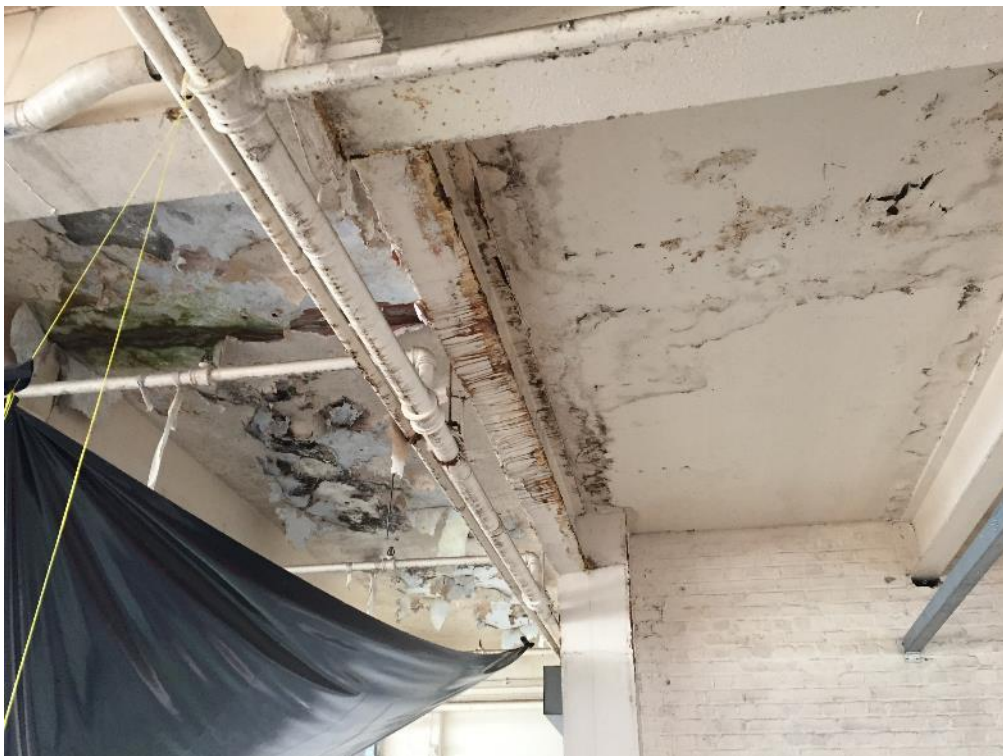
Photo 6: Original Building Condition
