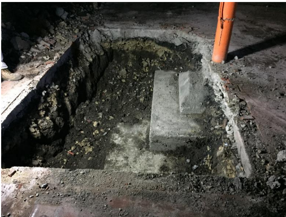
Photo 30: Tiered spread footing
