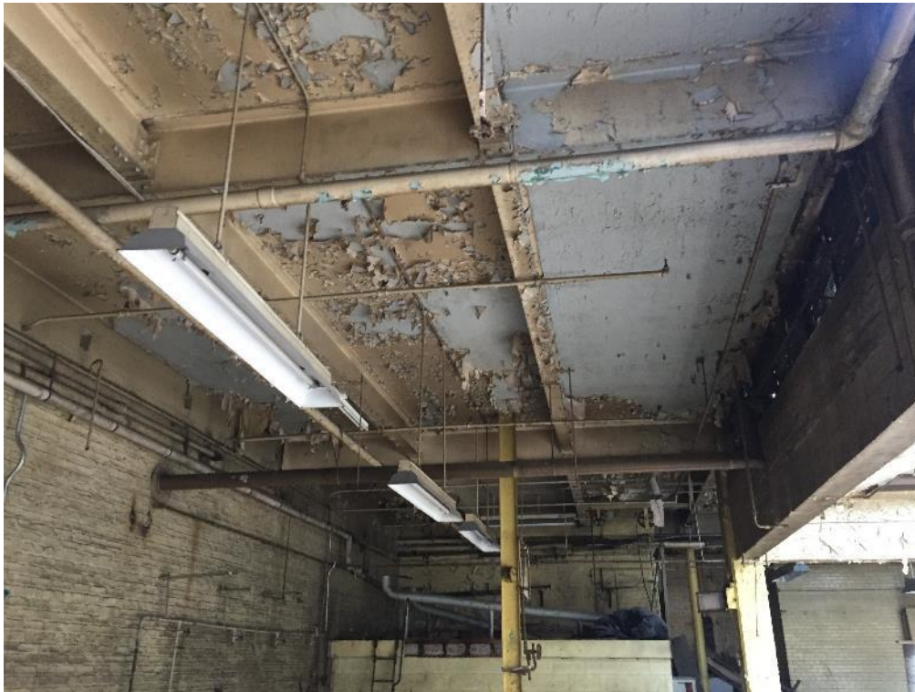
Photo 1: Original Building Condition
