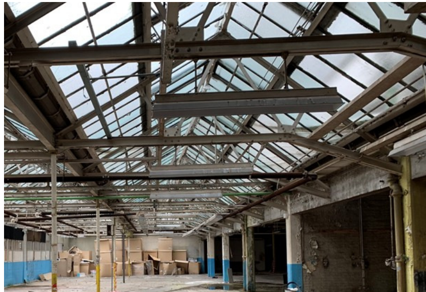
Plate 5: Steel roof trusses
