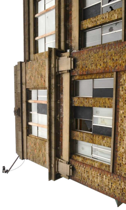
5. View of the western bay of the front façade of Block A
