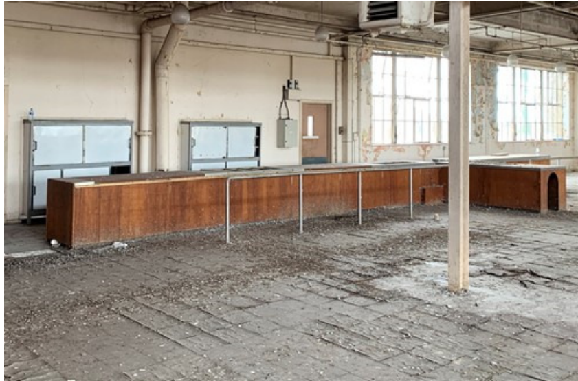
Plate 12: Kitchen equipment and counters
