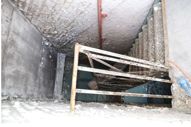
10. View down staircase at R3
