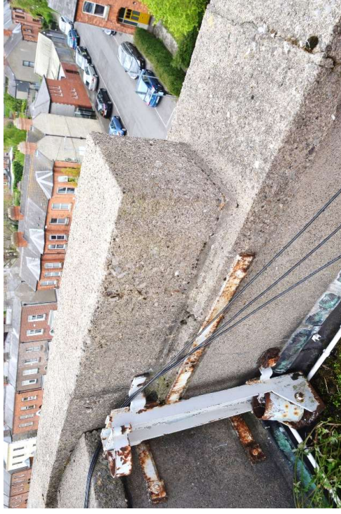
18. View of the rear of the front parapet wall
