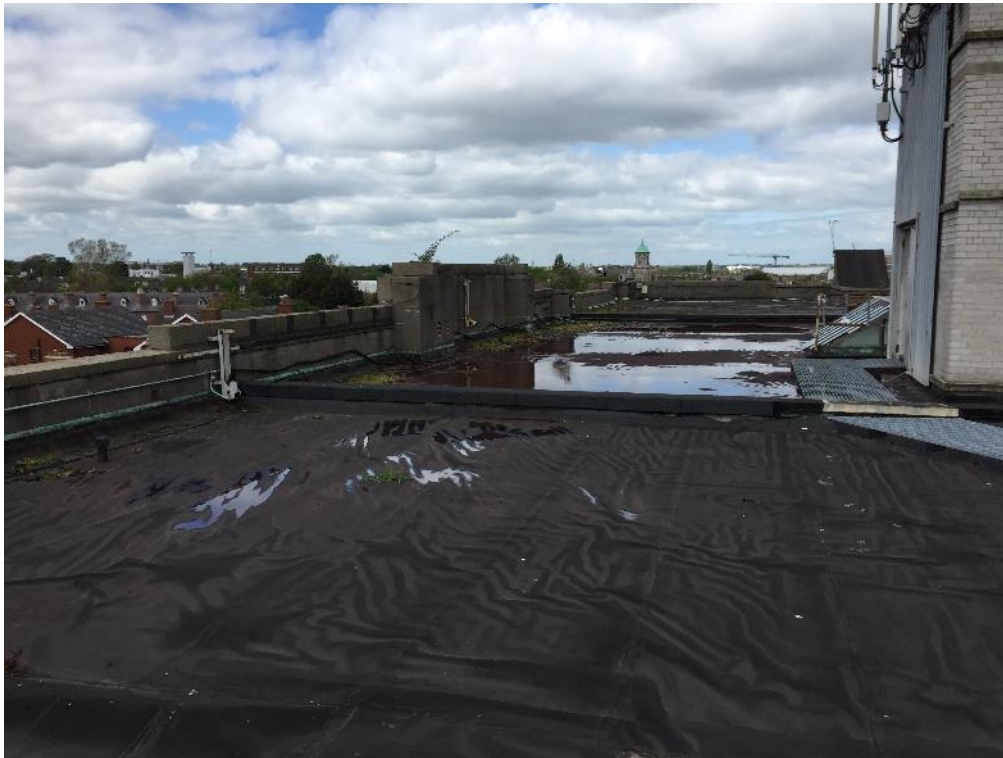
Photo 10: Original Building Condition
