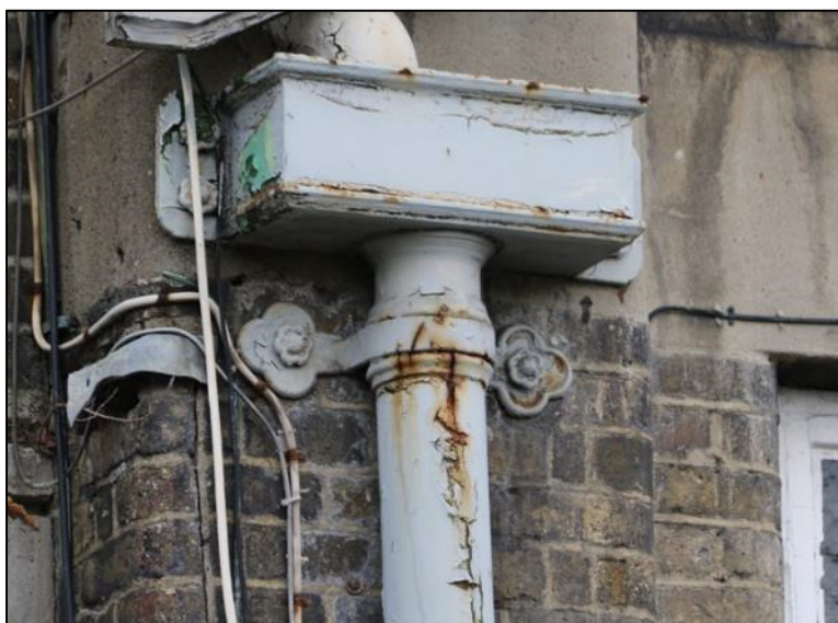
Plate 2: Rainwater hopper, downpipe and strap
