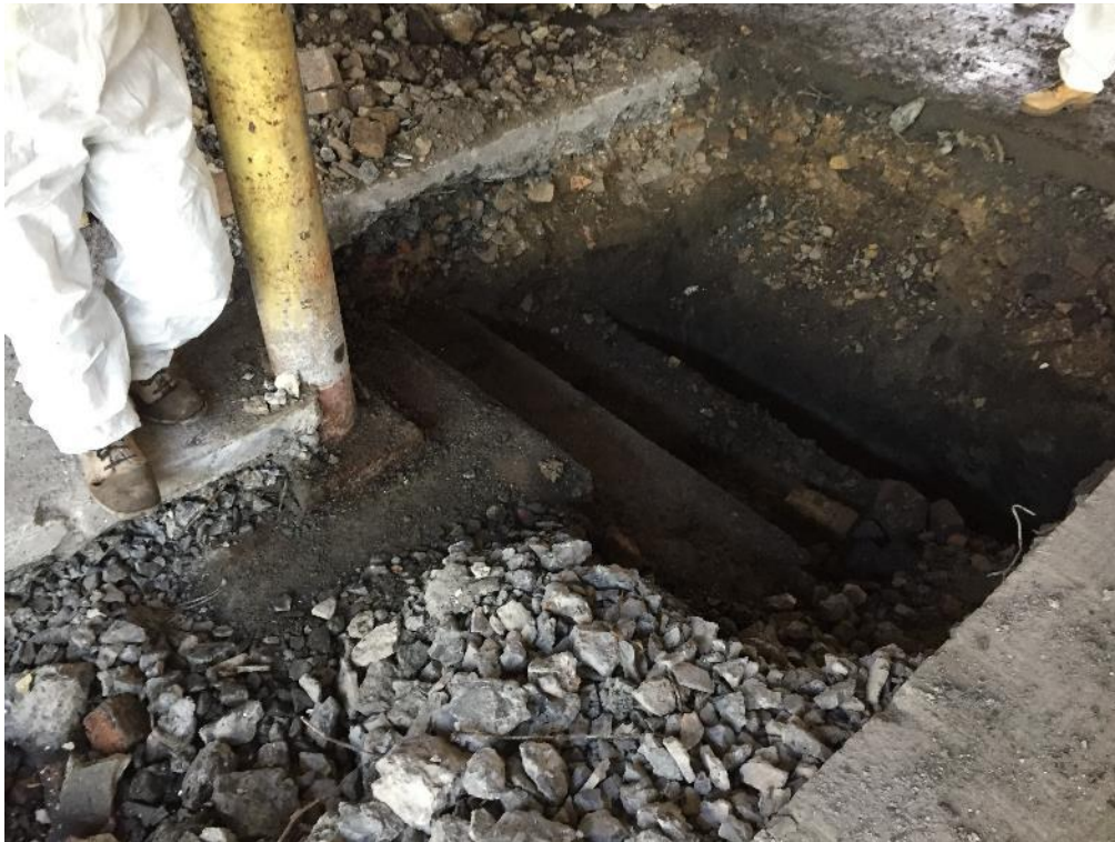
Photo 31: Tiered spread footing
