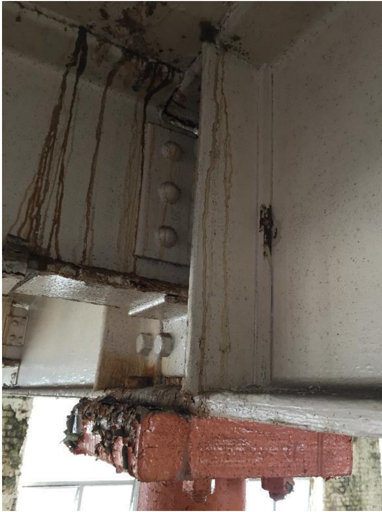
Photo 12: Typical column head connection
