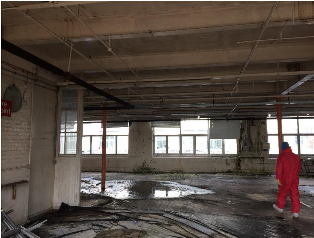
Photo 3: Original Building Condition
