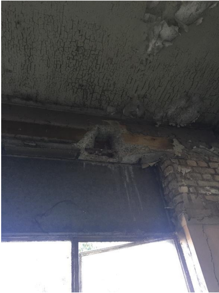
Photo 17: Embedded Steel
