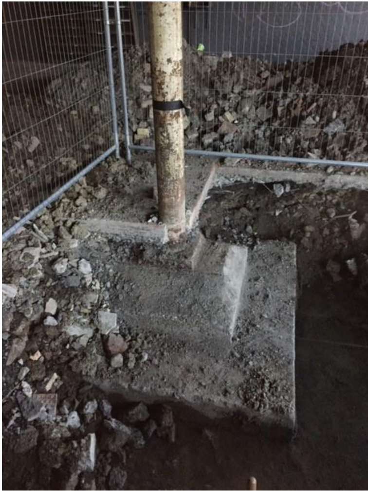
Photo 28: Tiered spread footing
