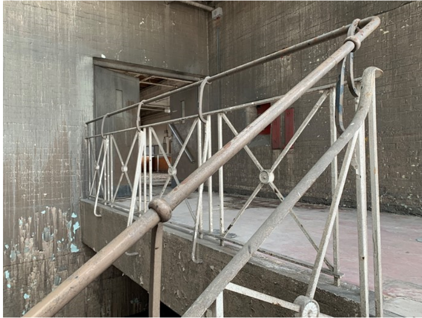
Plate 8: Wrought-iron railings on staircase
