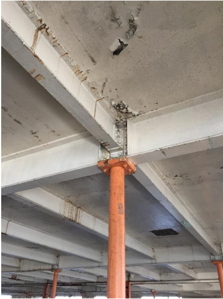
Photo 11: Typical Ground/First Column and beam
