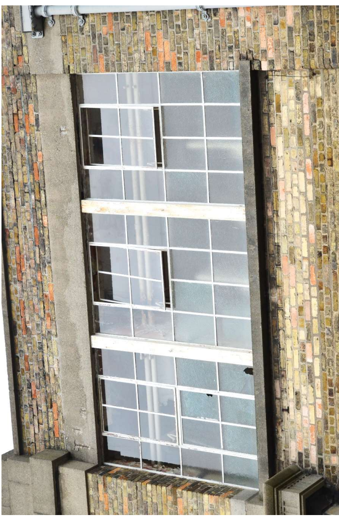
27. Original multi-pane window at the later 1930s level of Block A
