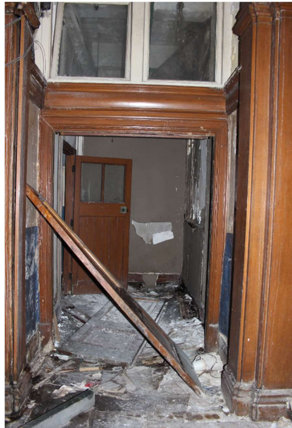
Figure 4: View of internal joinery elements within the front three bays of factory No. 2, including architraves, skirtings and timber panelling.
