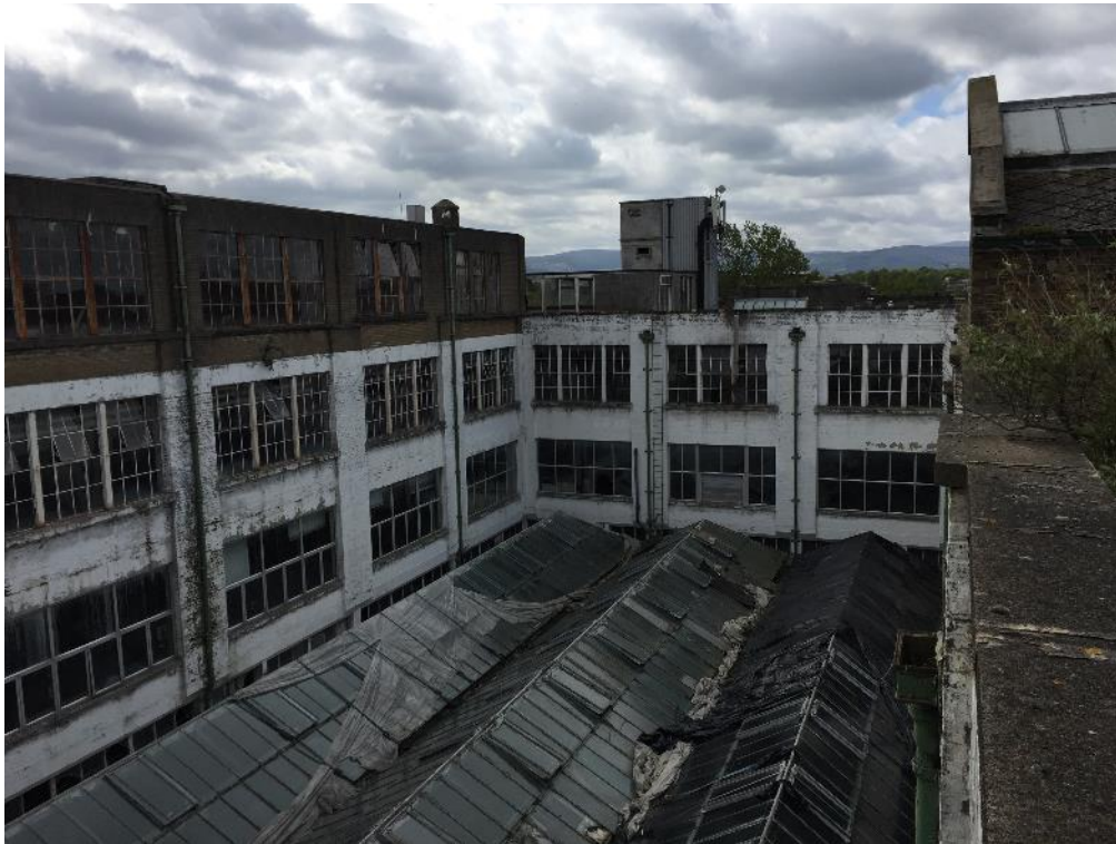
Photo 8: Original Building Condition
