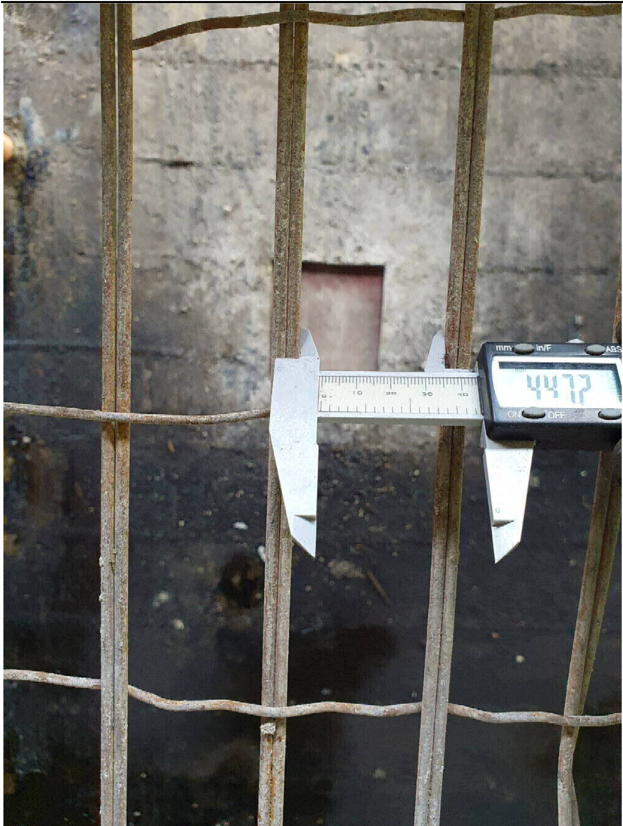
Slab Reinforcing Steel
