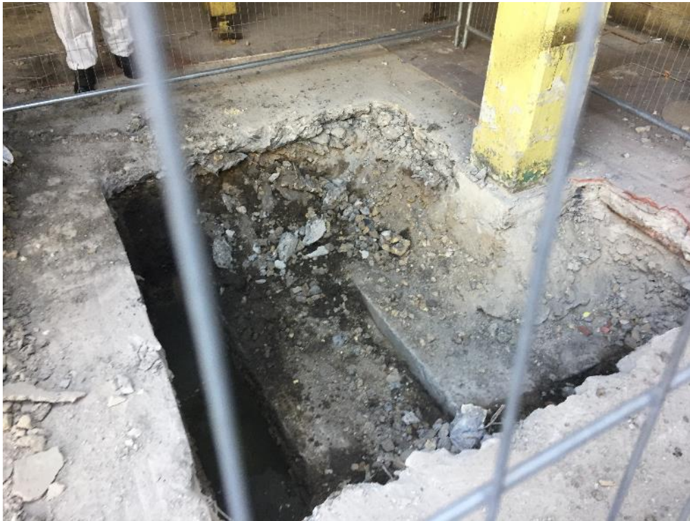
Photo 29: Tiered spread footing
