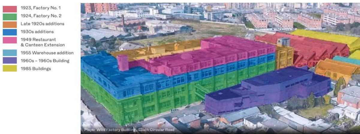
Figure 1.1 – Player Wills Factory – Construction Stages.
