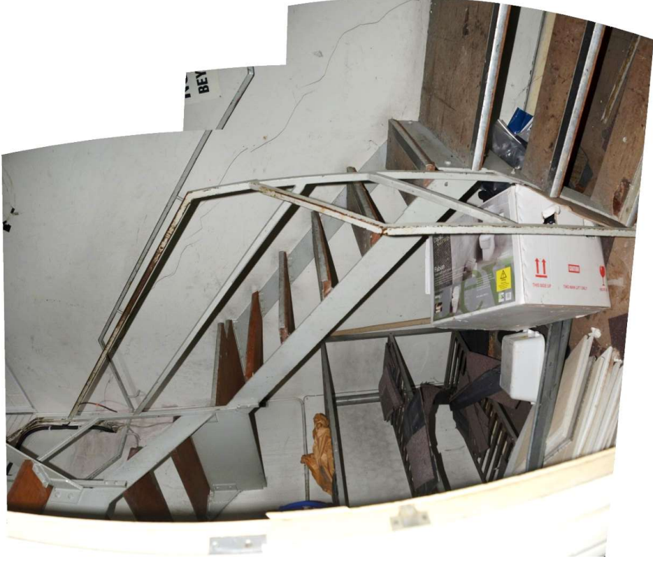
30. Stair Hall – First Floor Level
