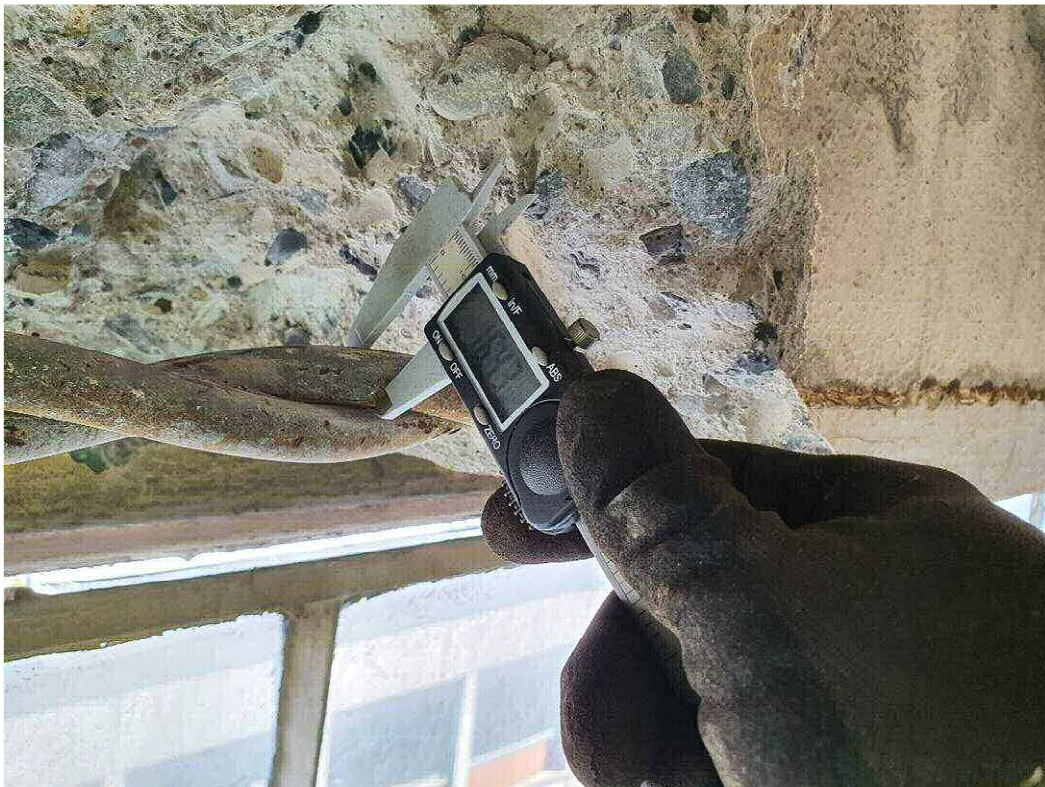
Beam above windows reinforcing steel
