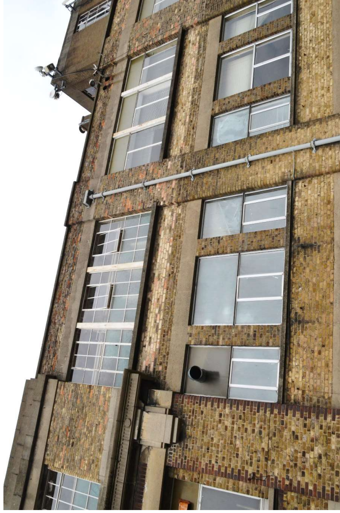
24. View of the junction between the original two-storey building and the 1930s second floor extension (Block A)
