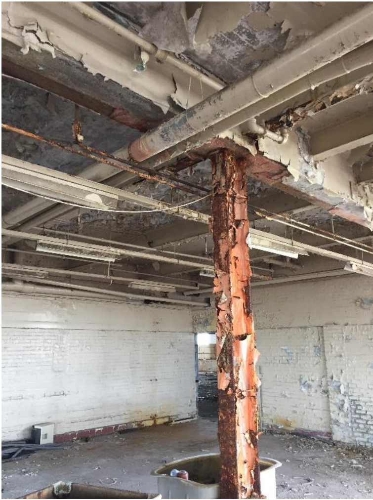
Photo 7: Original Building Condition
