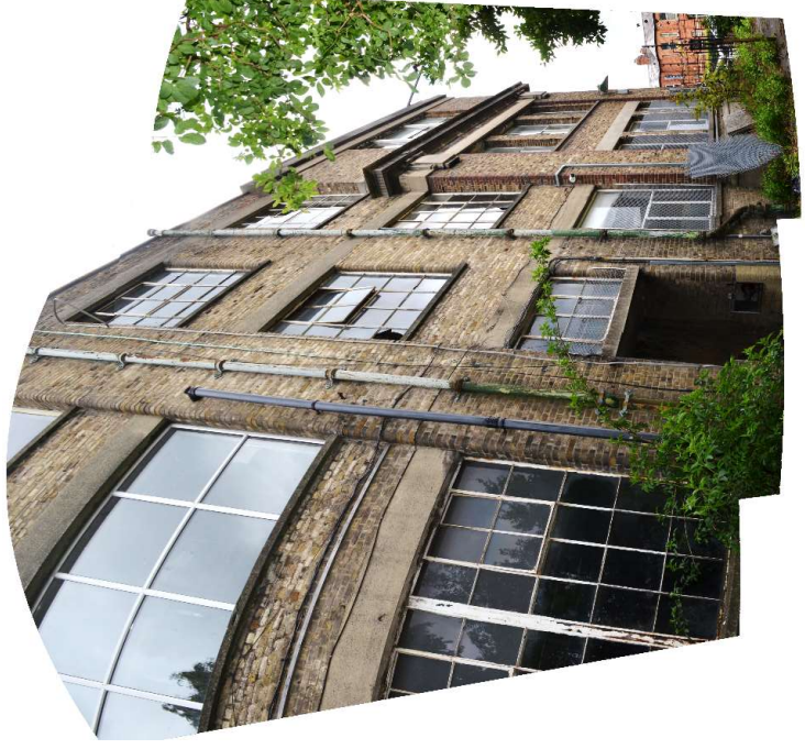
61. Oblique view along the western elevation of Block A
