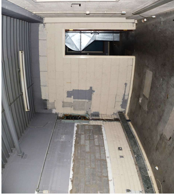
51. Storage Space – Attic Level
